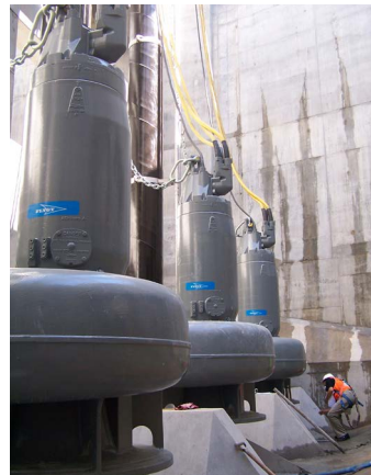
Height-adjustable and rotatable cast-iron stand for dry vertically installed pumps (10-100kW)
